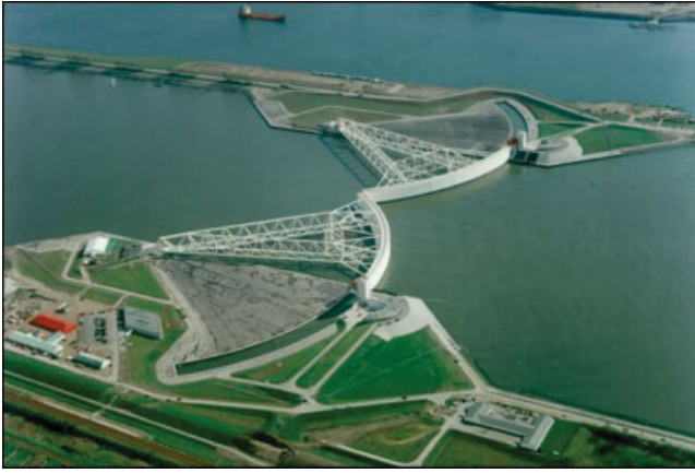
FIG. 1. View on the Maeslant storm surge barrier [1]. [Color figure can be viewed in the online issue, which is available at www.interscience.wiley.com .]
